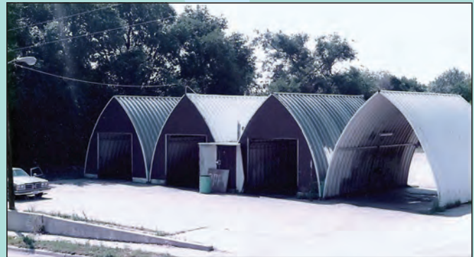
The car wash formerly at 6901 Mercy Rd. in Omaha.
